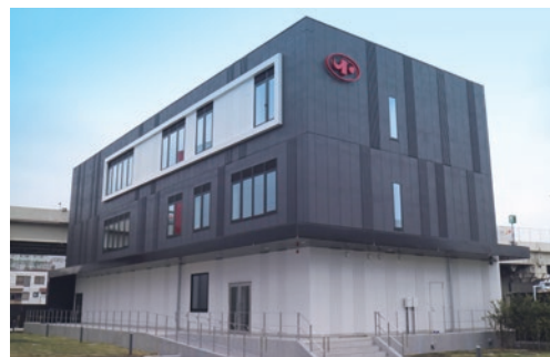
Yokohama Mirai HRD Yokohama Mirai HRD is a specialized facility for human resource development at Yokorei. There are rooms to accommodate large groups, along with smaller training classrooms. The facility is also equipped as a system development center, allowing for large-scale software development to support future strategic ICT investments.
