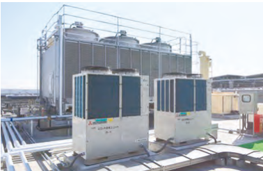
Refrigeration equipment that uses CO2 alone
