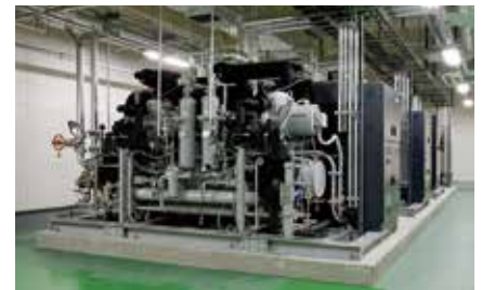
高効率自然冷媒冷凍機 Highly efficient natural refrigerant air conditioning system
