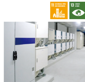
Storage cells at the Kesenuma Sorting Spot
